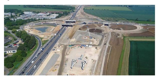
**Section 6:** Preparatory works continue here. Completion of archaeological investigations on Mill Common has allowedutility companies to start protecting or diverting their assets in this area. On the west side of Huntingdon, top soil stripping has begun and a Virgin Media asset has been installed.
