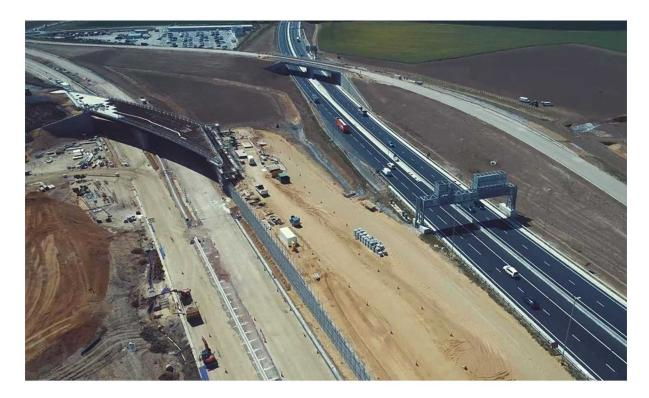
**Section 3:** Mainline surfacing of the Huntingdon southern bypass is progressing well and should be completed in late summer. Surfacing on the bridge over the East Coast Mainline railway is complete, allowing site access to Brampton. Highway communications works are well underway with ducting and gantry installation continuing across the section.
